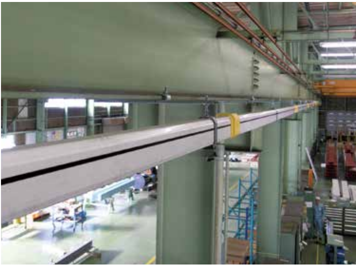
Installation example of traveling electrical supply rail
